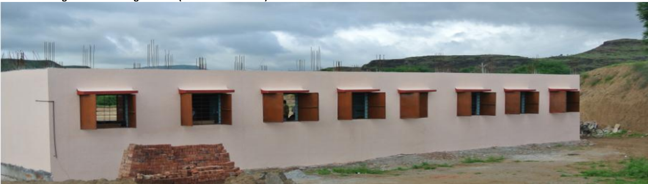
School Building- Back side- August 2014
