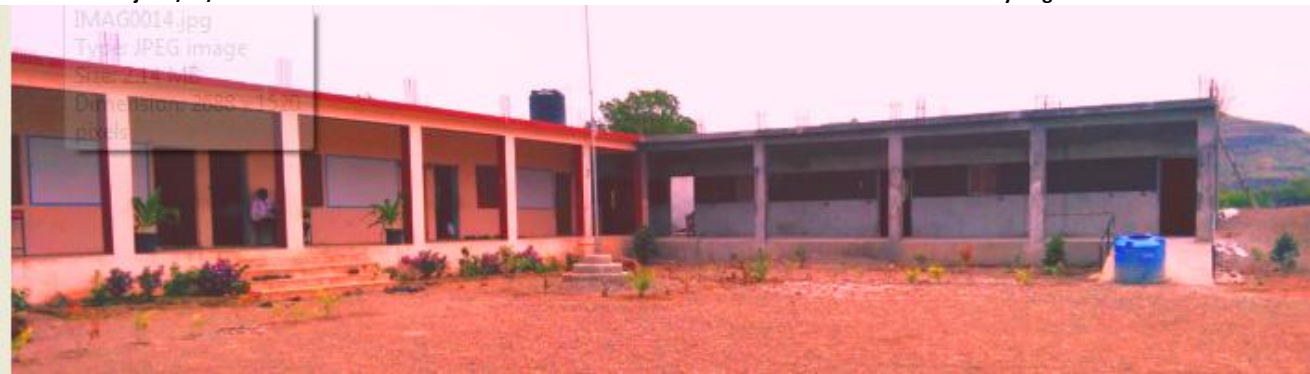
School Building- Front side- August 2014 (six class room Built)
